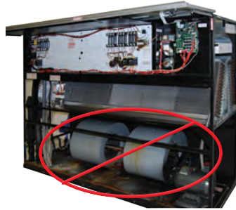
Eliminate the inefficient centrifugal blowers
