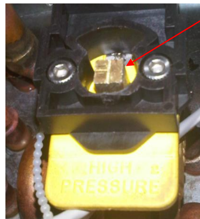
Valve Stem Marking
