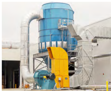
Dust Collection System
