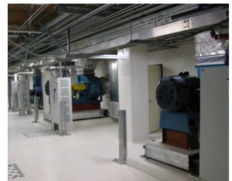
Exhaust Fans for Nuclear Plant
