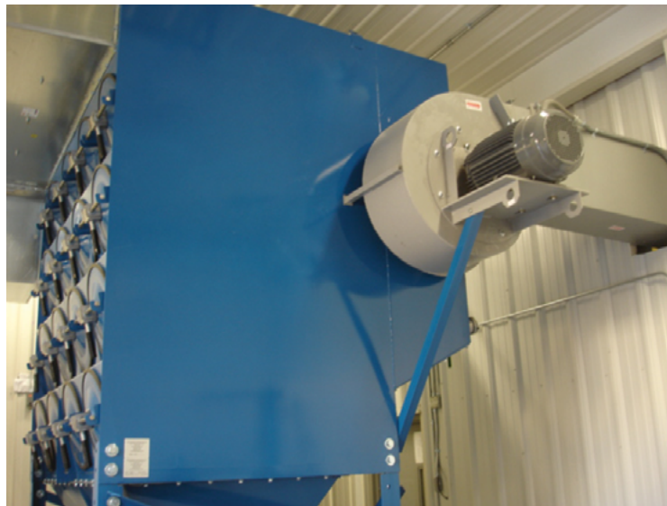
Arrangement 4HI (horizontal, inlet mounted) on a cartridge-style dust collector (support by customer).
