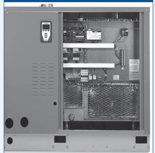
Figure 7-2: View of keypad, subpanel and cleanout plate
